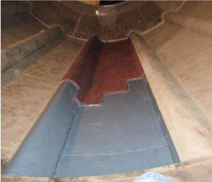
Belzona 1811 (Ceramic Carbide) is a two-component repair and protective coating for the protection of surfaces subject to abrasive attack.
