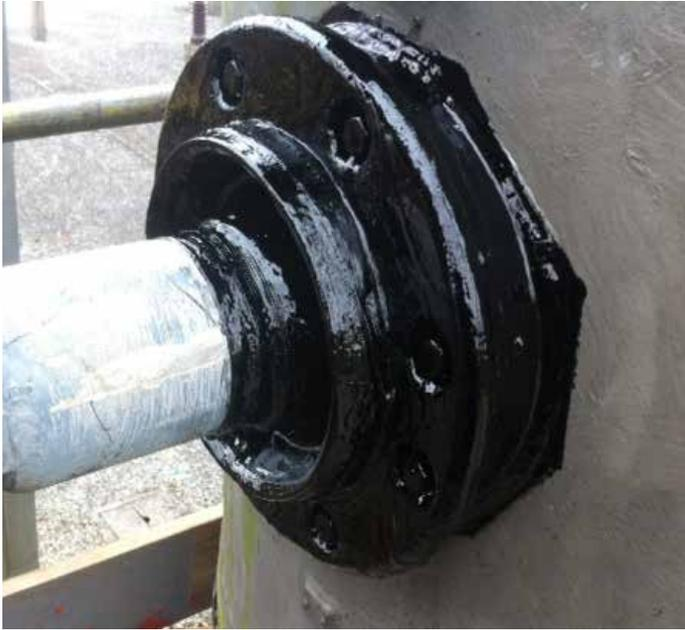
Belzona 2111 (D&A Hi-Build Elastomer) is a two component, elastomeric material designed for repairing, rebuilding or creating rubber components.
