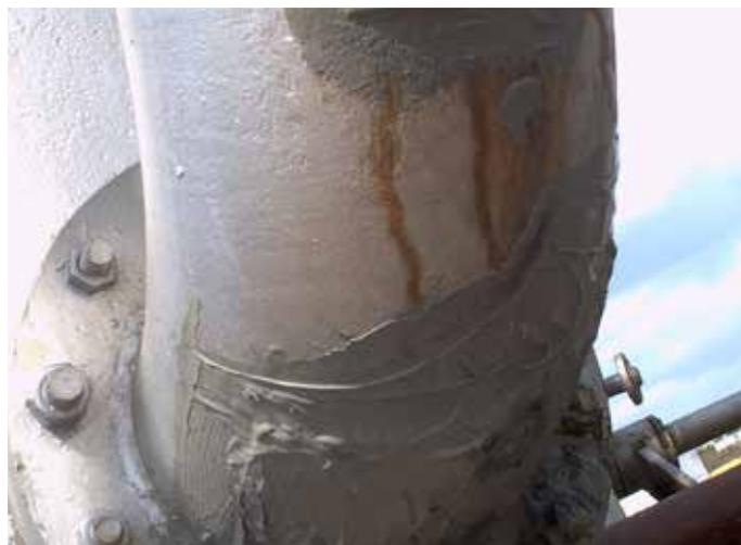
Belzona 4301 used to bond plates to pipes suffering from chemical attack
