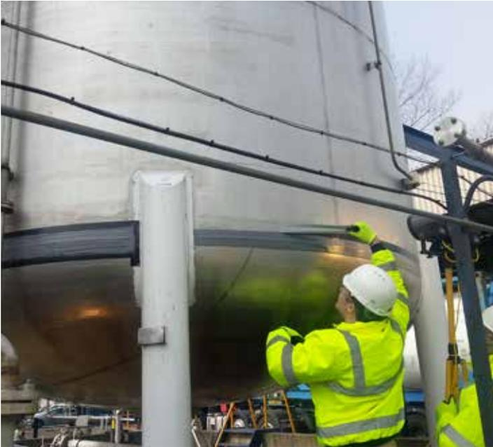
Belzona 4301 (Magma CR1 Hi-Build) is a high performance, paste-grade system with outstanding chemical resistance to a broad range of chemicals. This material is designed for rebuilding or protecting metal and concrete surfaces against chemical attack. In addition, it is ideally suited to repairing damaged chemical resistant linings.
