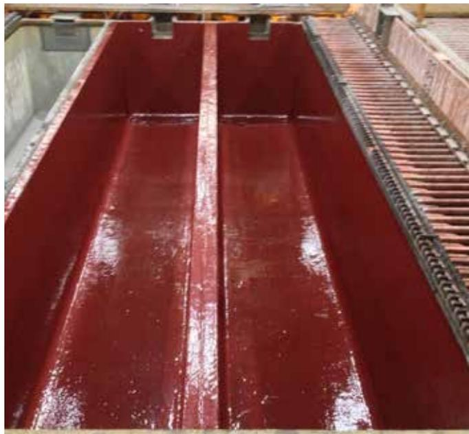
Belzona 4341 (Magma CR4) is a two-component barrier coating for protecting surfaces subject to chemical attack. It is optimised for resistance to inorganic acids, such as sulphuric and hydrochloric acid, up to 90°C (194°F).
