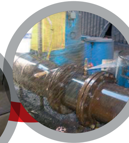
Sealing Leaking Pipes
